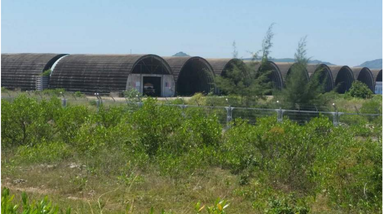
Old Chu Lai Hangars
