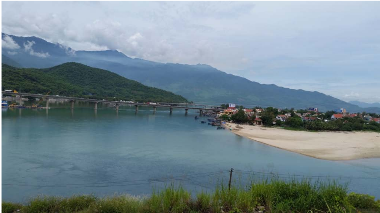
Bridge at the north end of Hai Van Pass into Lang Co
