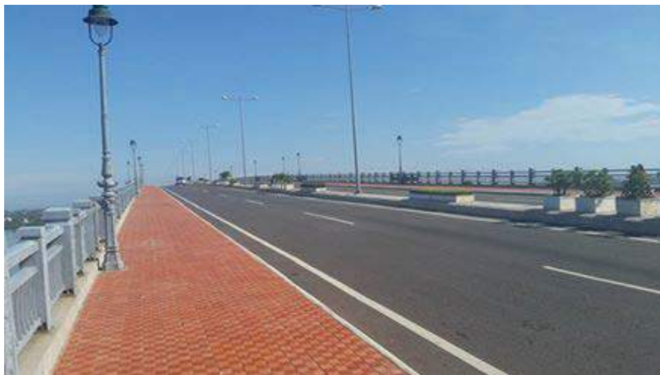
New Cua Dai Bridge at Cam Thanh on New Highway South from Hoi An
