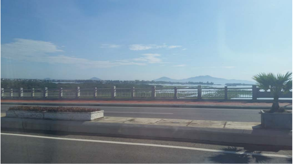
View from New Bridge
