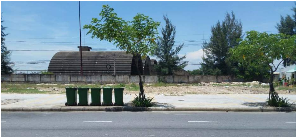
Old Hangars at Marble Mountain Air Facility
