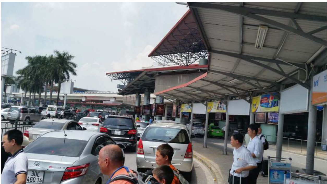
Ha Noi International Airport
