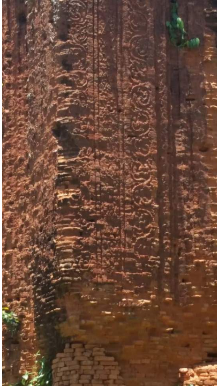
Khong My Towers Brickwork
